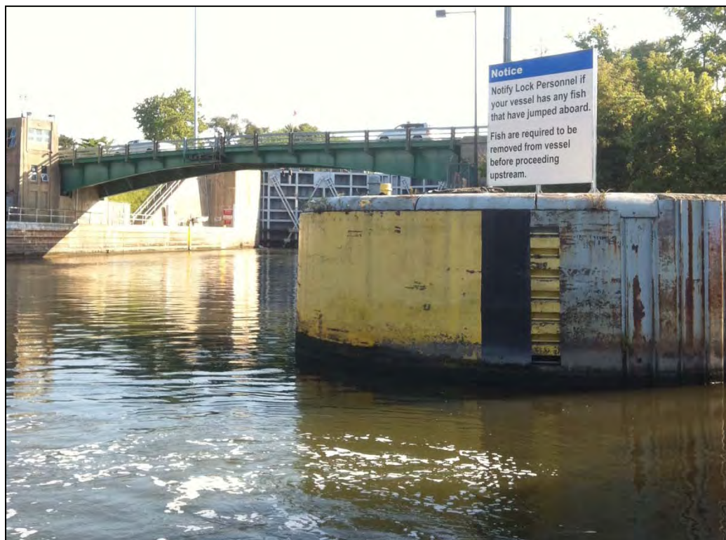
Figure 2.14 Photo of signage installed at Brandon Road Lock and Dam
