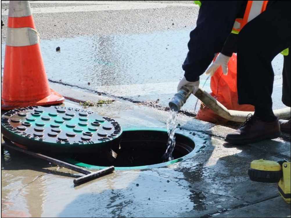
Exhibit 3. Hose from fire hydrant flushing sewer
