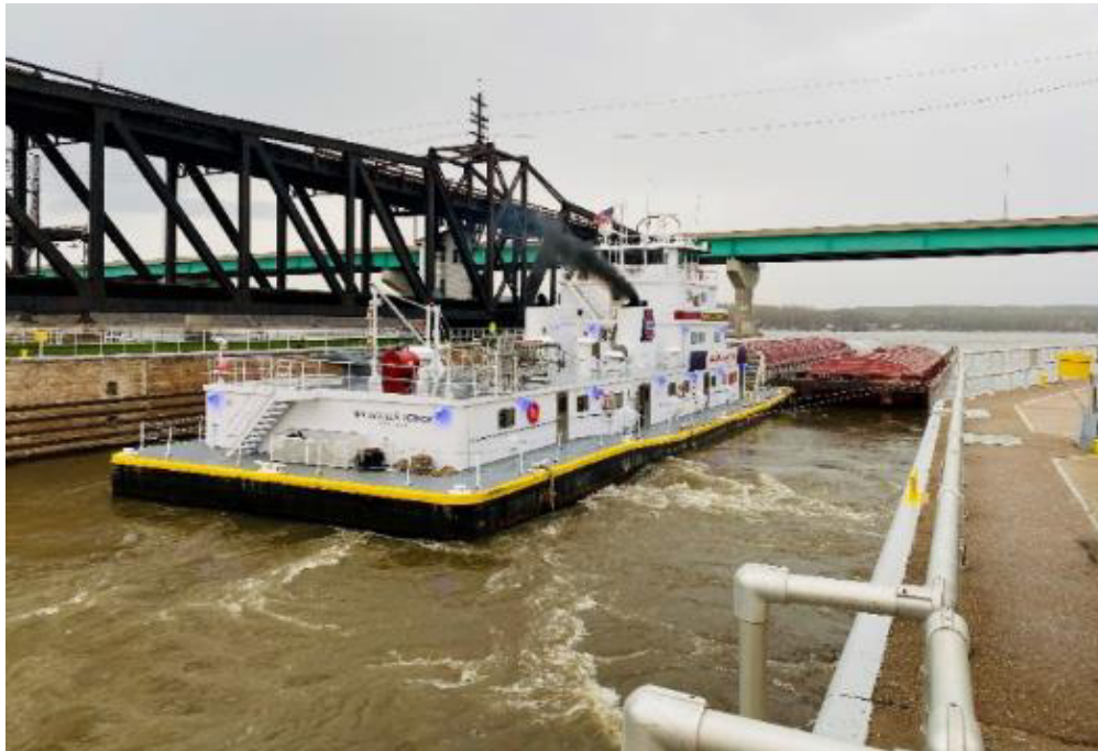
Figure 16 — Downbound Tow Traversing uADS – Lock 19 (Keokuk, Iowa)
