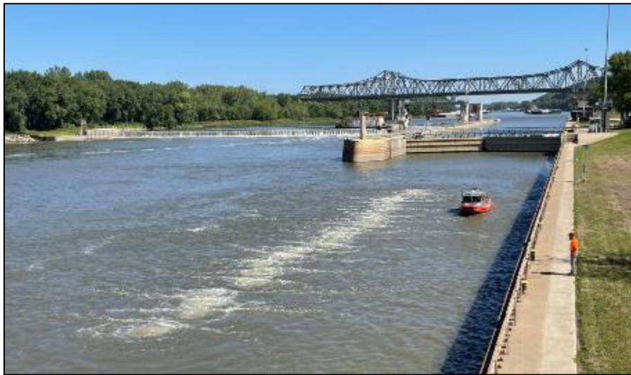
Figure B-5 — ABC Deterrent Prototype in Operation at Peoria Lock and Dam
