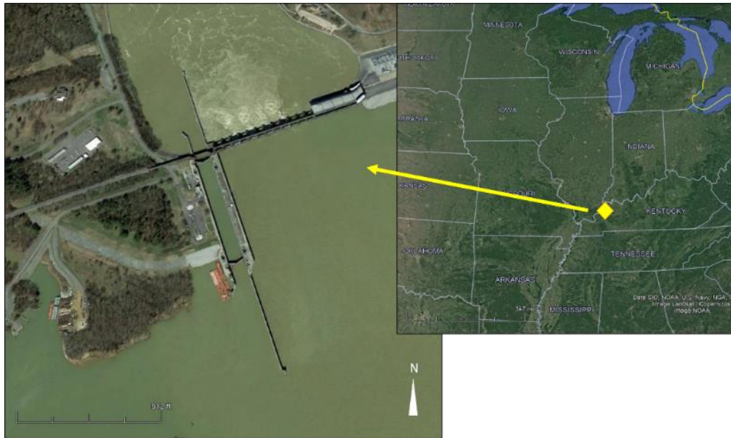
Figure 35. Barkley Lock and Dam on the Cumberland River near Grand Rivers, Kentucky
