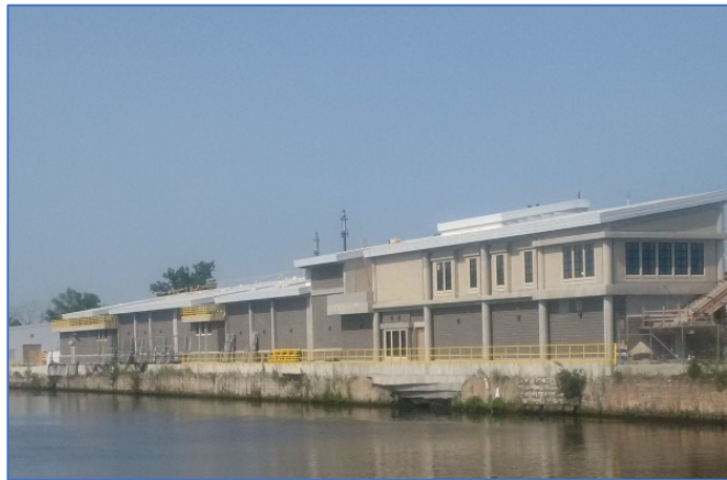
Permanent Barrier I. Photo Credit: USACE
