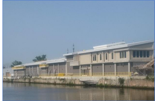
Permanent Barrier I. Photo credit: USACE
